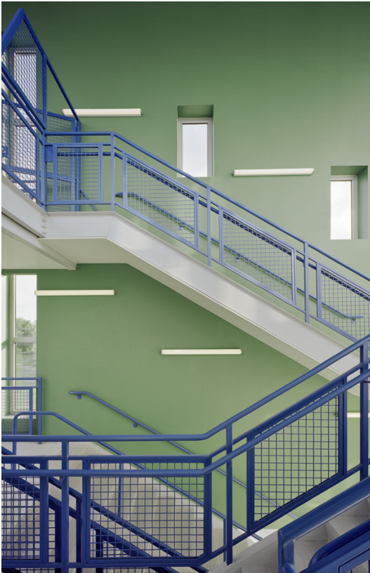
Byram Hills School District | Crittenden Campus Photo courtesy of Perkins Eastman | Photographer: Paul Rivera/ArchPhoto
